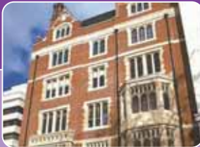
Conference and Training Facilities, Arundel House, London
